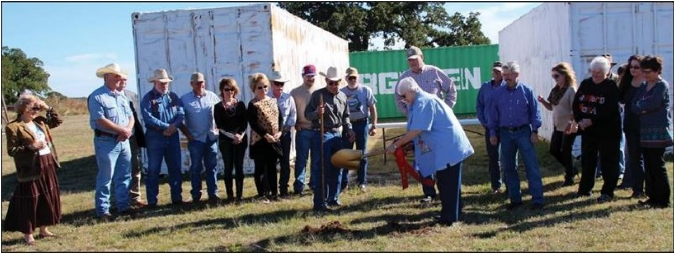
Groundbreaking was made by Milta Carter on October 31st, 2014 to start construction on our Tales 'n' Trails 9,200 square foot Agricultural Center.
